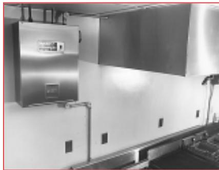
**Simple to install, easy to service.** The design of the Ansul R-102 System features simplified piping and nozzle placement. And thanks to its cartridge operation, the Ansul R-102 System is reliable and can be recharged faster on site than stored pressure systems. All of which means a more flexible, efficient system that can be installed easier and with less disruption to your facility.
